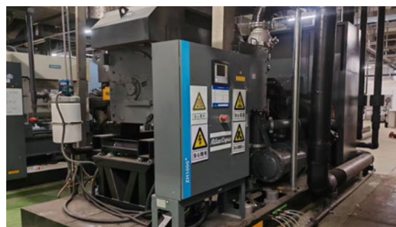
Air Compressor Energy-Saving Retrofit
